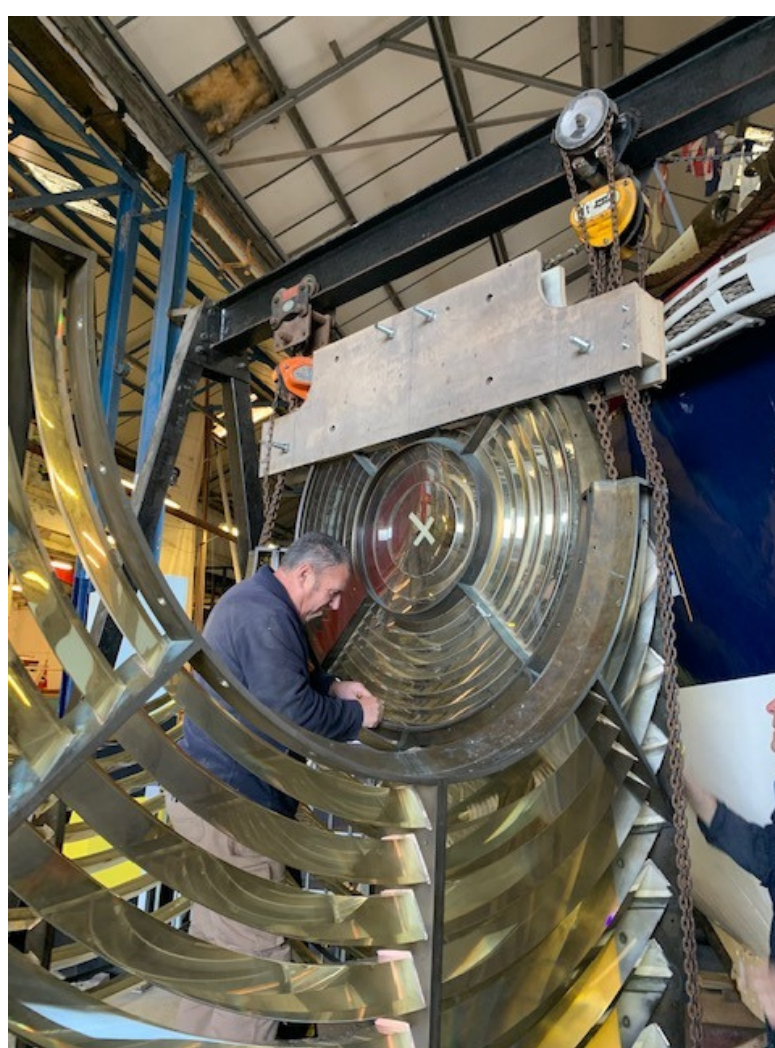
The volunteer team working to rebuild the lens and the completed lens in The Boat Shed
